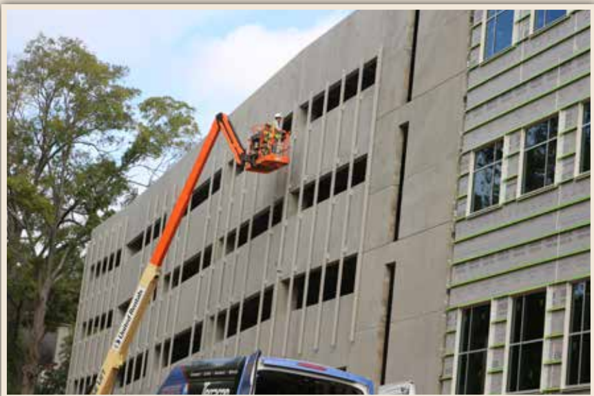
Grids have been installed to assist with installation and the mounting of metal panels.
