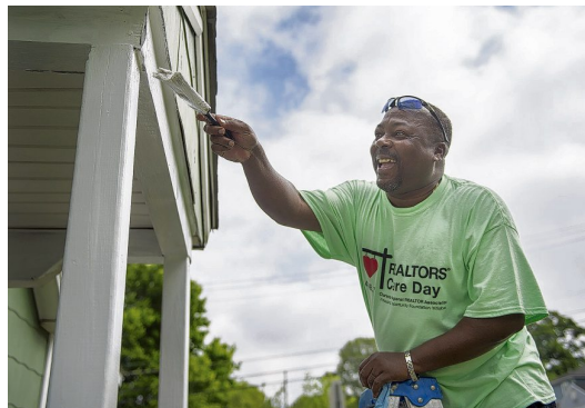
Jernel Sanders smiles as he helps paint the front porch of a house on Double Oaks Road.
